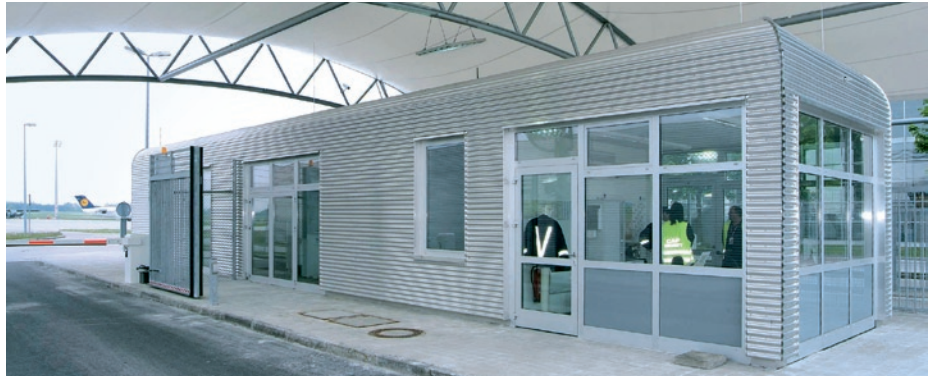
Car checkpoint with corrugated aluminium cladding, lighting system and diaphragm roof.
